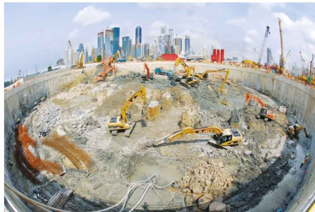
■ Excavation in 120m diameter circular cofferdam
