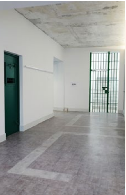
■ Traces of detention cells found on the ceiling and ground floor slab of Block B
